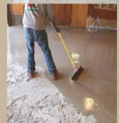
Leveling Mortar
