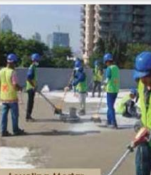
Leveling Mortar
